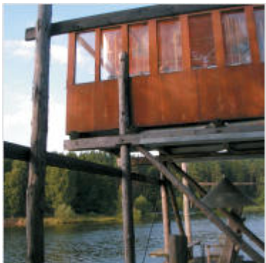
95 Degrees A staggered series of platforms, supported by a network of wooden scaffolding, gives the 95 Degrees restaurant a slightly tilted cantilever over the Klyazma Reservoir. Photo by Yuri Palmin/courtesy Alexander Brodsky and Oleg Ovsvy
