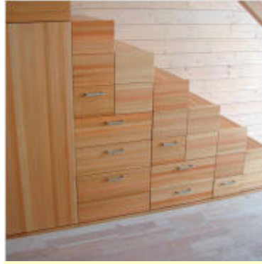
Brodsky also designed the house's built-in staircase drawers. Photo by Mark Lamster
