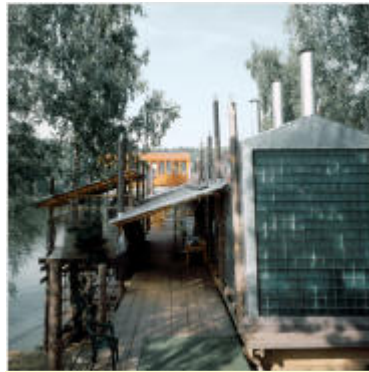
The structure was built based on Brodsky's sketches rather than on formal building plans, and has an estimated area of 3,700 square feet, including open terraces, a covered pavilion, and a glass-and-galvanized steel kitchen. Photo by Mark Lamster
